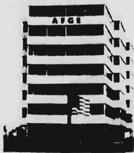
J. F. GRINER BUILDING
